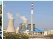
Coal fired power plant
