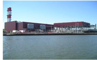
IPP(US: Astoria I gas power plant)
