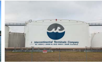
US: tank terminal for chemical products
