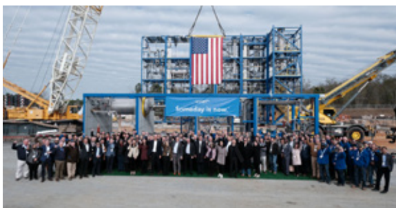
LanzaJet demo-plant in the US (under construction)
